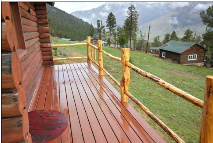
New porch on Foose cabin.
